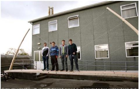
Cable stayed bridge with elegantly tapered, curved glue-laminated pylons and box beam deck
