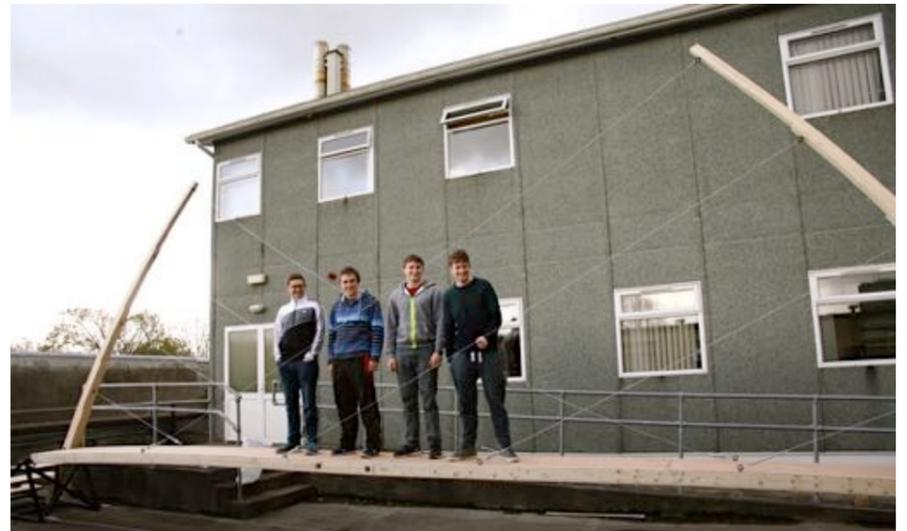
Cable stayed bridge with elegantly tapered, curved glue-laminated pylons and box beam deck
