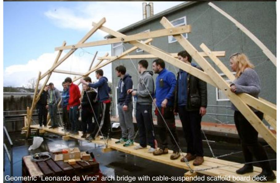
Geometric "Leonardo da Vinci" arch bridge with cable-suspended scaffold board deck
