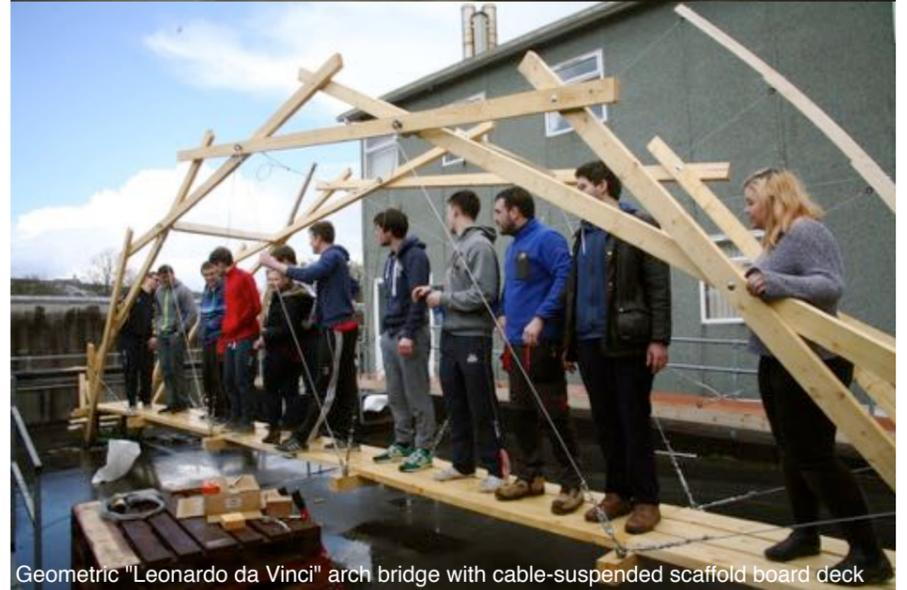
Geometric "Leonardo da Vinci" arch bridge with cable-suspended scaffold board deck
